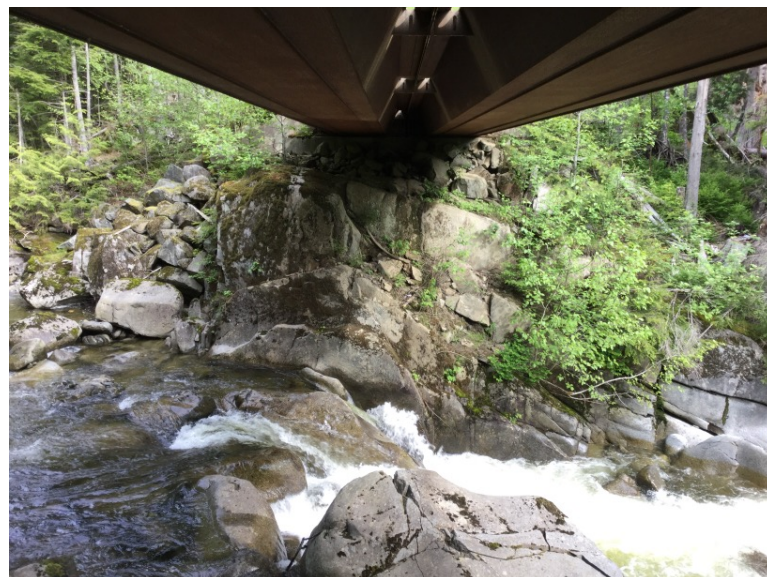
Left Bank Abutment when facing downstream
