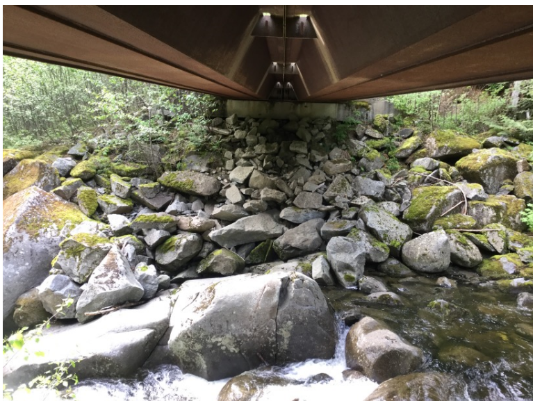
Right Bank Abutment when facing downstream
